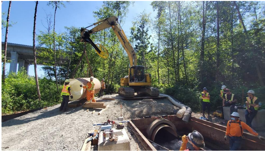
Figure 4 - an insertion pit with next pipe ready to go in.
