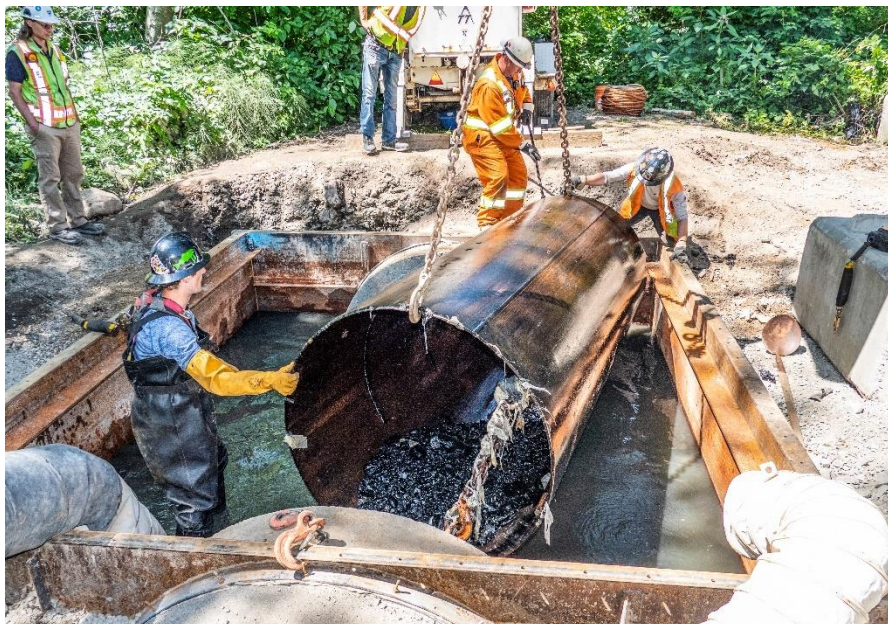
Figure 3 - Dredging and debris removal
