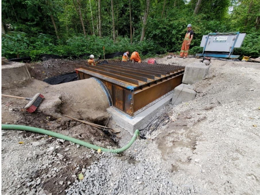
Figure 2 - Water tight flow control chamber with lid that can be removed or replaced in under 30 minutes.
