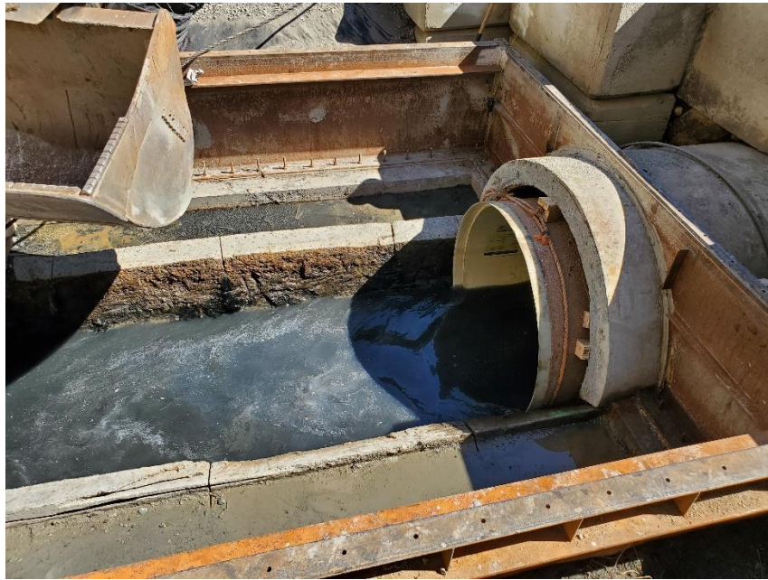
Figure 5 - The new liner in place during a moderate flow
